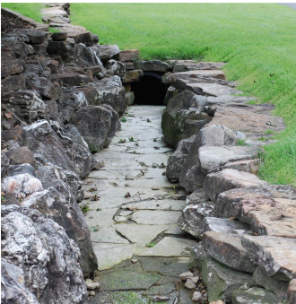
Dry creek bed — boulders and creek rock carry the runoff
