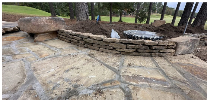
Boulder bench — slab seat on stone piers at the fountain
