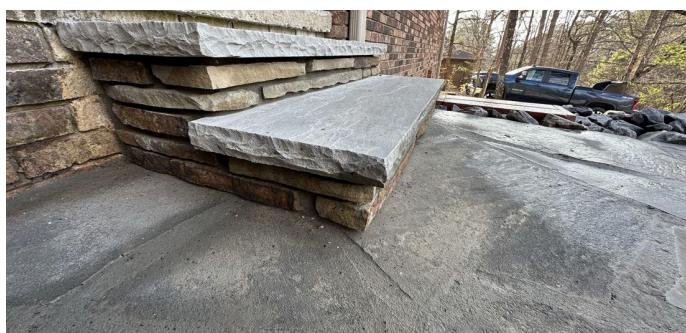
Slab step — at the patio edge
