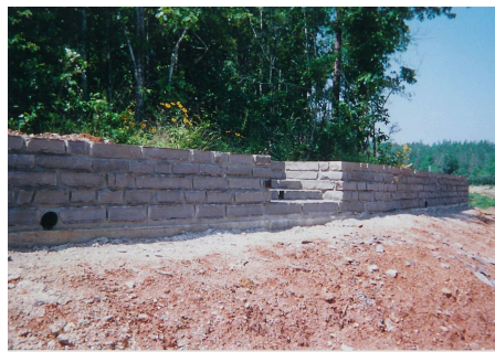
New chopped-stone wall — before the backfill
