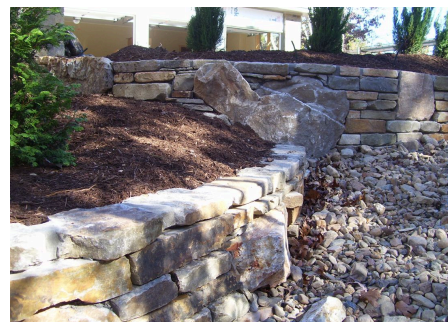
Stacked wall — over creek rock
