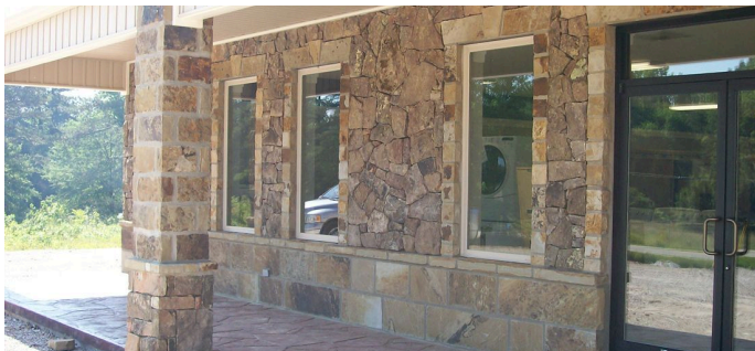
Storefront columns — close
