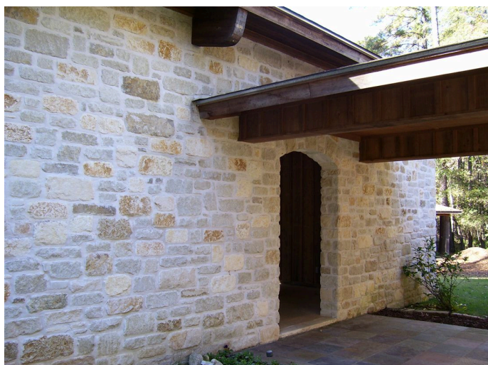
Cream limestone — wall and doorway
