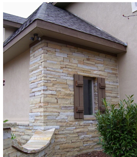
Dry-stack wall corner — lantern post
