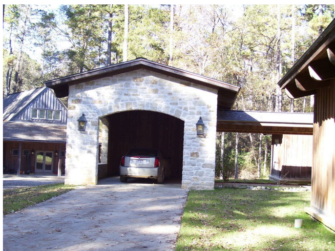
Limestone porte-cochere — timber roof
