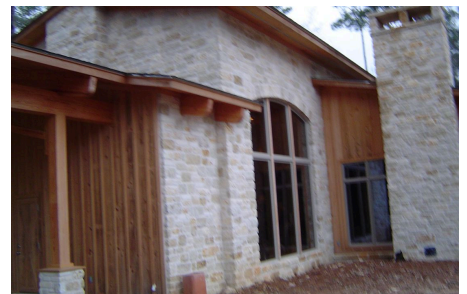
Gable end — limestone under the timber roof
