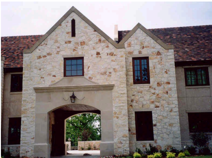
Cut limestone — porte-cochere
