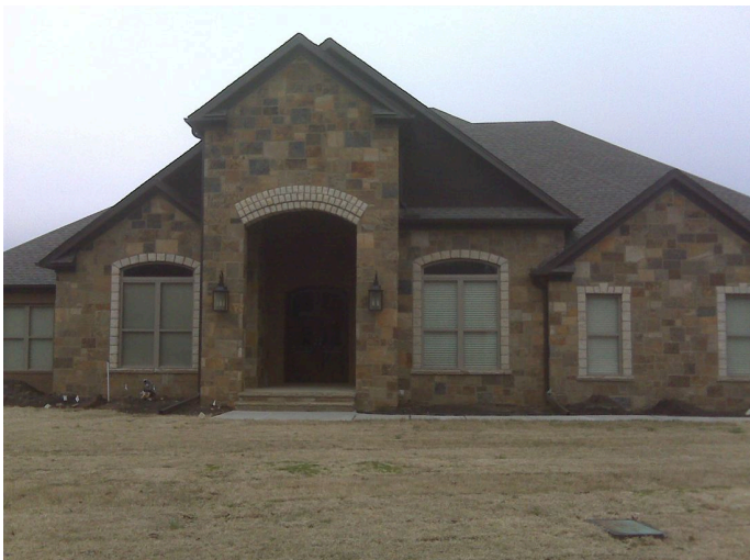
Chopped stone and stucco — arched entry
