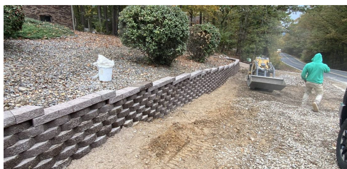
Garden retaining wall — segmental block along the road
