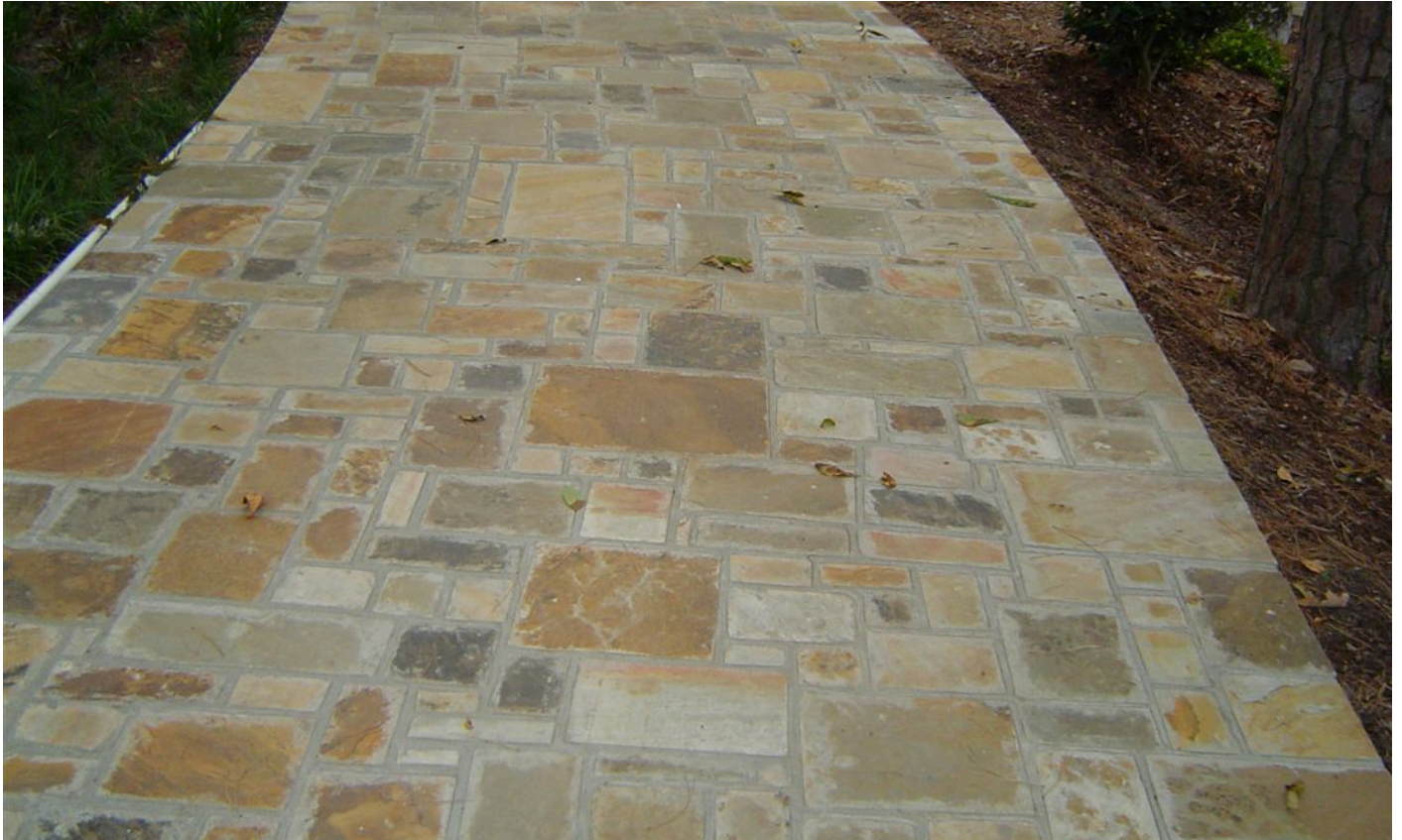
Oklahoma flagstone walkway — ashlar pattern
