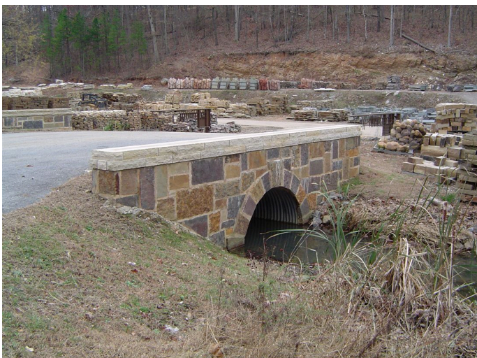
Culvert headwall — and truck entrance
