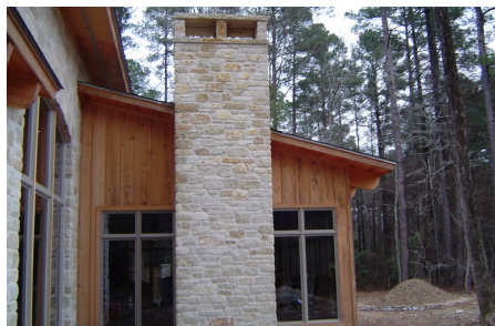
Chimney — full-height cut limestone
