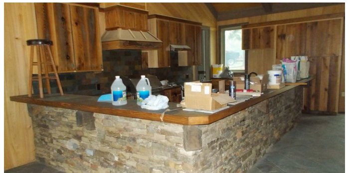
Kitchen island — stone base
