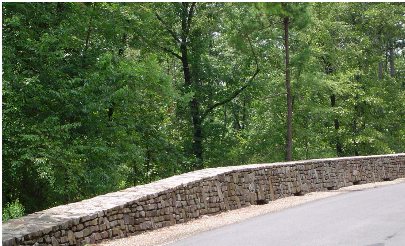
Road wall at the bridge — curved dry-stack ledge stone with a cut cap
