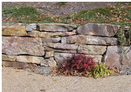
Low garden wall — dry-stack sandstone
