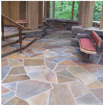
Cut-slab steps with copper rail — flagstone landing
