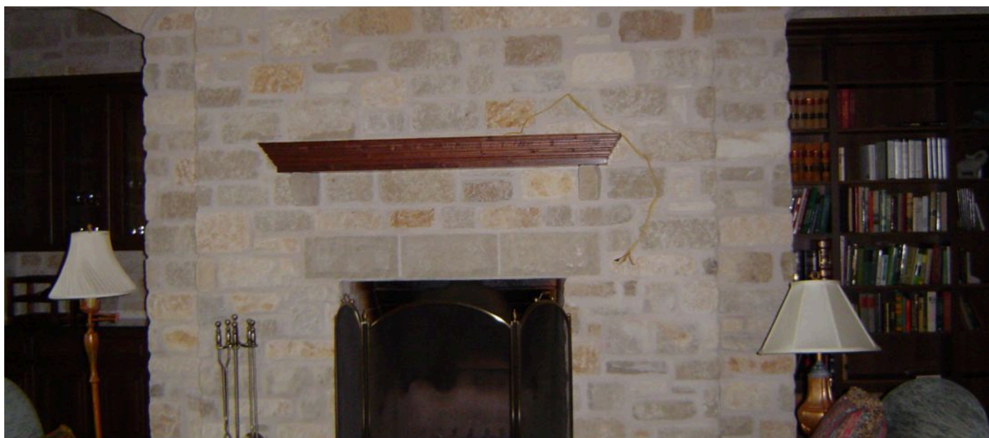
Fireplace wall — cut limestone between the bookcases, timber mantel
