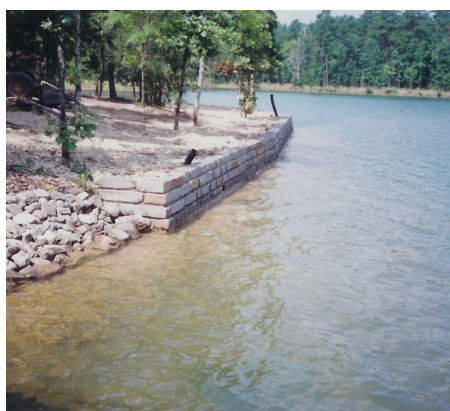
Stone seawall — with riprap
