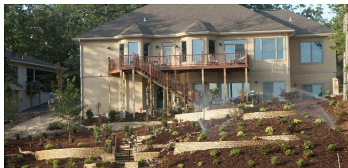
Terraced walls — on a lake slope
