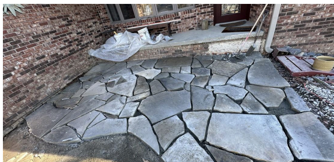
Setting the flagstone — over the old concrete slab
