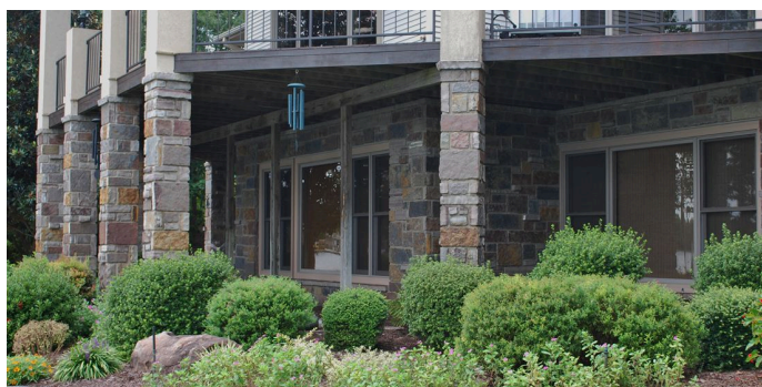
Stone-column house — layered foundation beds
