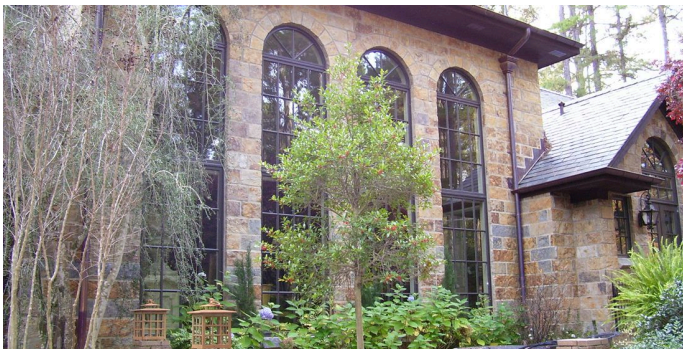
Courtyard elevation — arched windows
