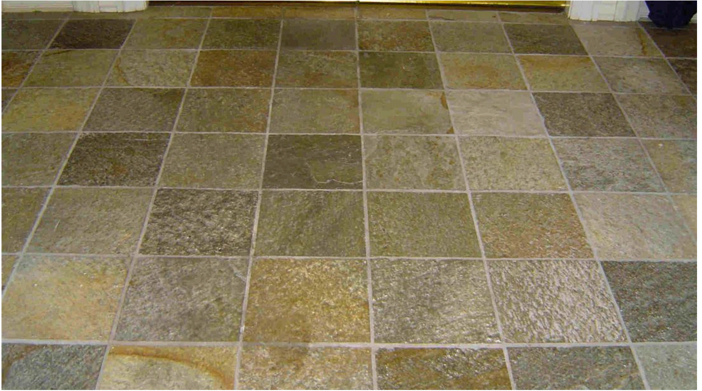
Quartzite tile floor — clubhouse
