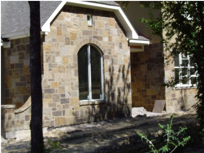
Stone house — arched window
