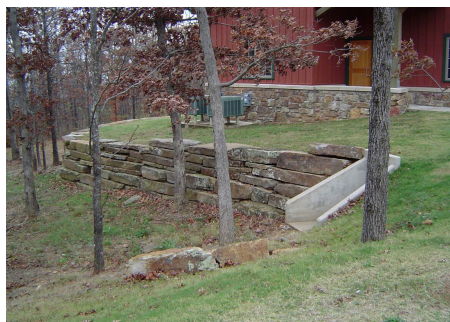
Stacked slab walls — at a farmhouse
