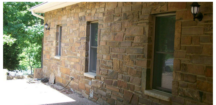
Chopped stone — exterior wall and door
