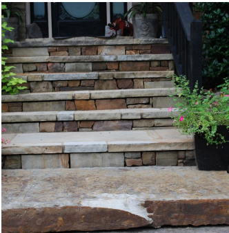
Front steps — ledge stone and slab treads
