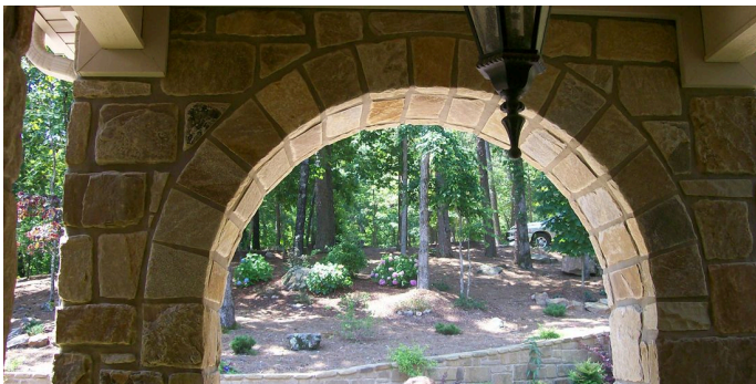
Interior stone arch
