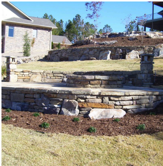
Curved seat wall — stone columns at the patio
