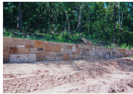
Chopped stone — the same wall from the road
