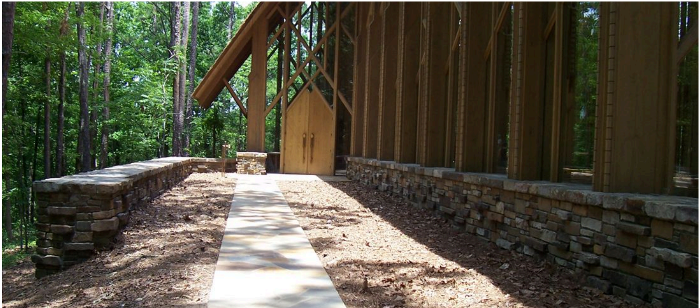
The chapel from the approach — flagstone walk, dry-stack seat walls and the stone base of the nave
