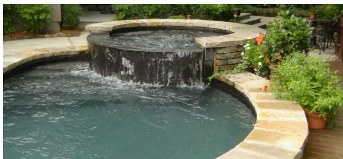
Raised spa — spillover into the pool
