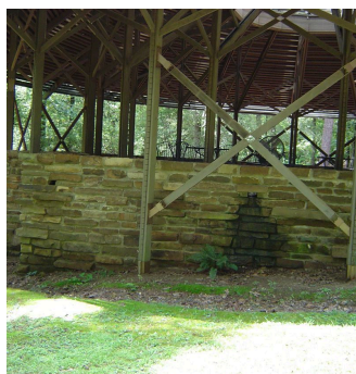
Pavilion — ledge-stone walls under the timber roof
